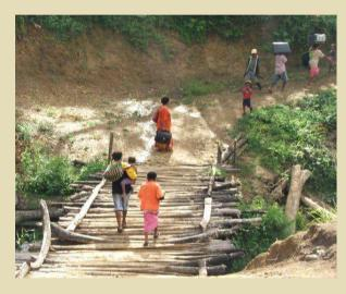
Locals built a log bridge in 2008. This bridge survived less than two years before flood damage and general degradation rendered it impassable to all but foot traffic, and less than 1 year more to become dangerous for pedestrians.
